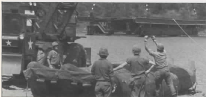
Division Engineers construct a float bridge across the Mississippi River
