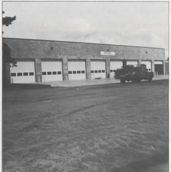
The new State Maintenance Facility, one example of more than $3 million in Federal construction at Camp Ripley during this biennium
