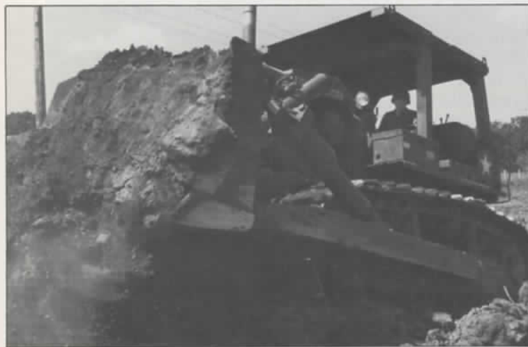
A Guard bulldozer levels ground for a park near Lake Elmo
