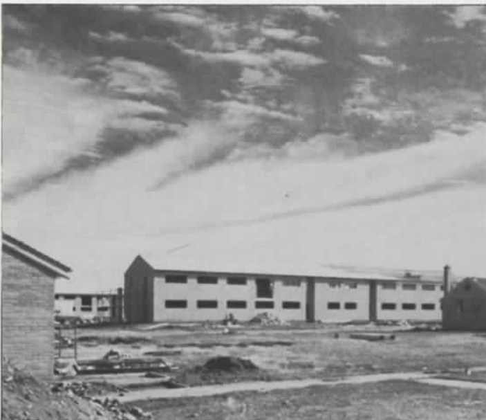
A seven-year winter barracks construction program ended during the biennium
