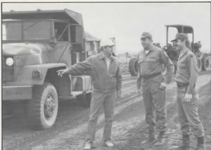
Guard engineers help construct a driver safety course at Dakota County
