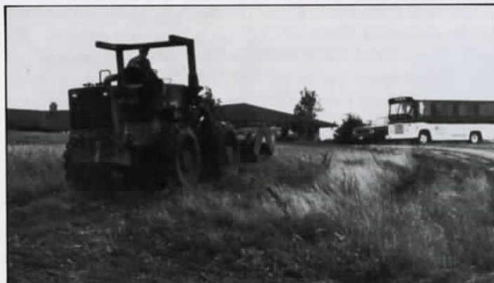
Engineers build nature trail at Vinland Center for handicapped
