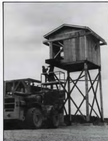
A new tank range tower at Camp Ripley.
