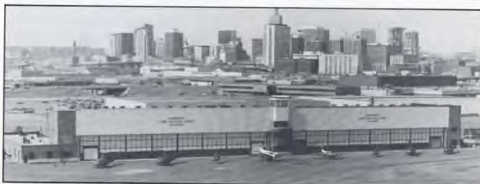
The newly-remodeled Army Aviation Support Facility (AASF) at the St. Paul Downtown Airport.
