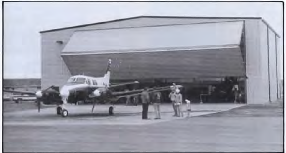
Camp Ripley's new aviation hangar.
