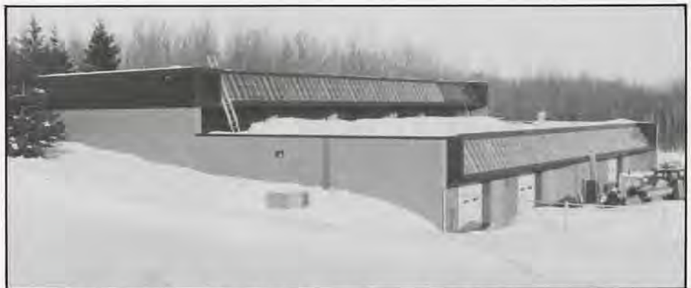
The weather outside may be frightful, but the energy bills for the new civil engineering building could be almost delightful, thanks to its solar panels.
