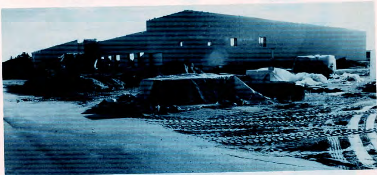
The Troop Issue Subsistence Activity at Camp Ripley, under construction
