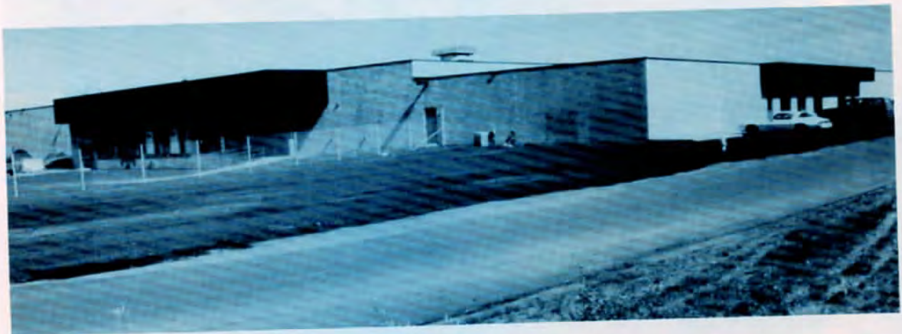
The USPFO warehouse at Camp Ripley
