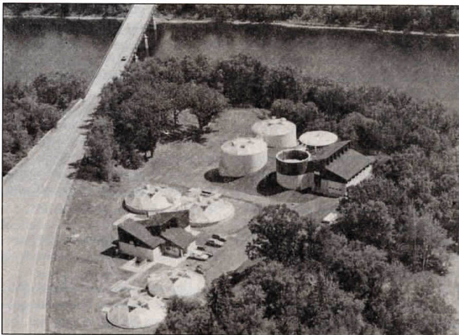
Camp Ripley received an award from the Minnesota Pollution Control Agency for exceptional compliance records in meeting water objectives during 1989 at the new wastewater treatment plant.
