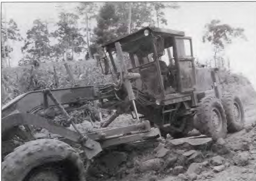
Soldiers of Company C, 142nd Engineers build a road in Panama.
